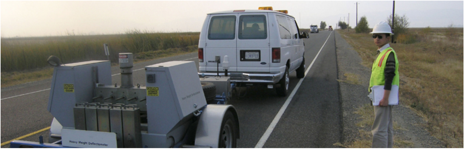
Pengcheng Fu at work on SR33 in Colusa County, the first Caltrans project using FDR-foamed asphalt
