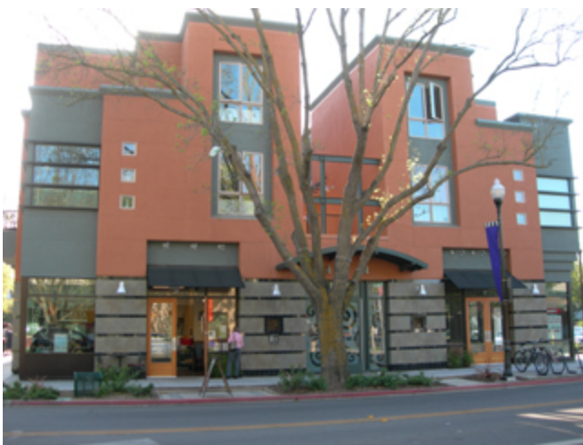
Example of ground floor retail with living space above Photo Credit: Dave Shpak
