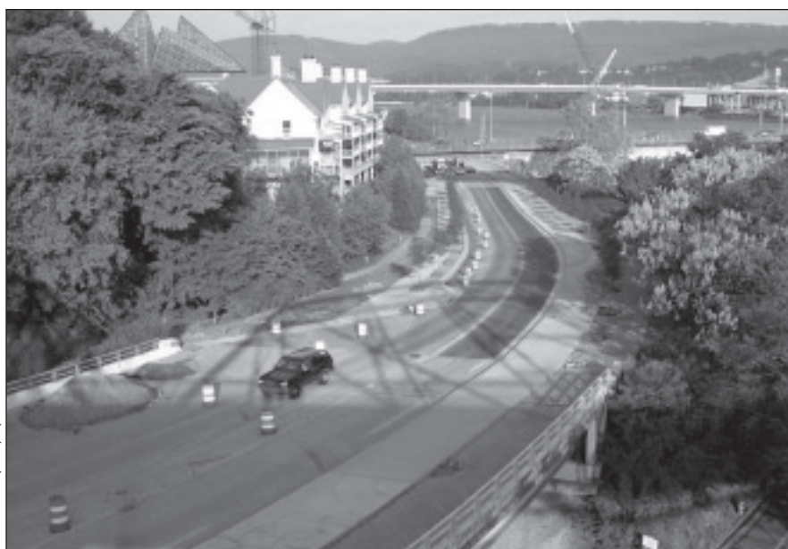
Figure 4. This construction photo shows the narrowing of the travelway and initial installation of one-sided on-street parking, walkways and street trees on Riverfront Parkway, Chattanooga, TN, USA.
